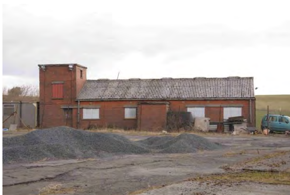
Photo 30: Building adjacent to barn at Photo 4
